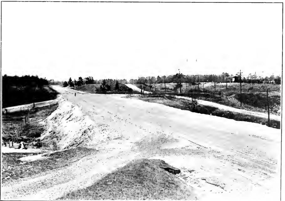
Grading, Middle Road, East of Credit Bridge.
